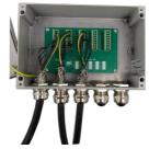
4. In the shelter, connect the 7G1.5mm<sup>2</sup> cable to the controller 113176-048. Use the cable through the M25 cable gland in the controller and set the switches.
