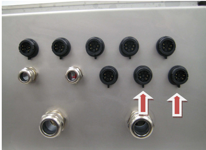
2-3-1-a: Position of the 8 connectors for each projector
