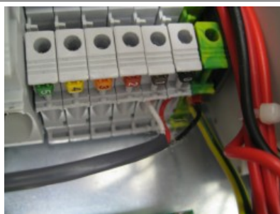
5. Wiring of the 3x1,5mm 2 cable from 24Vdc photocell on TB1 in the power cabinet
